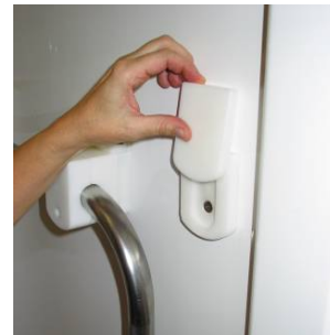
If the bar has to be removed, a cover plate can be installed.
